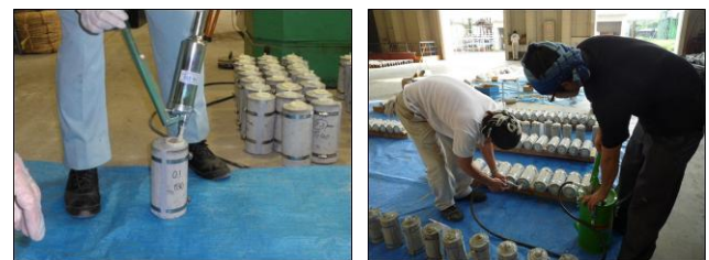
Fig.4 Injection of repairing material into concrete cracks
