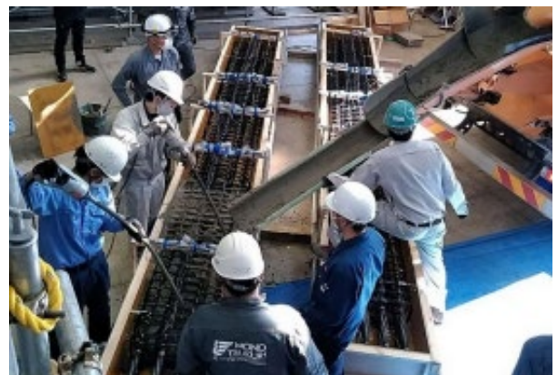
(b) Concrete casting
