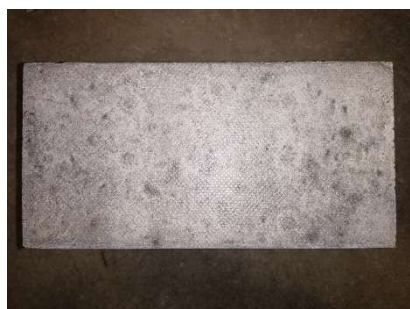
Fig. 10 Condition of top surface
