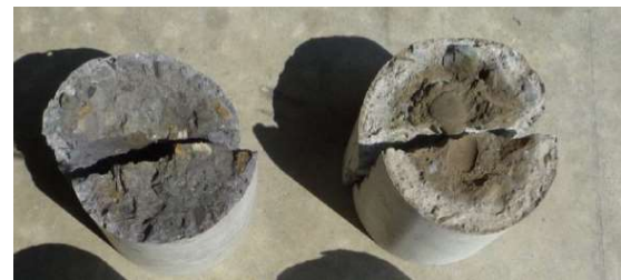
Discolored boundary by chloride ions
