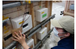
(h)断熱養生温度測定
