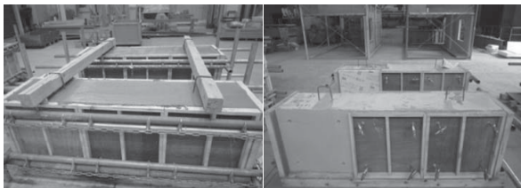
Placing of concrete Demolding at age of 1 day
